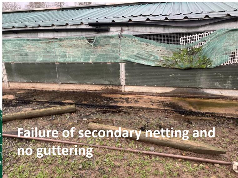
Failure of secondary netting and no guttering
