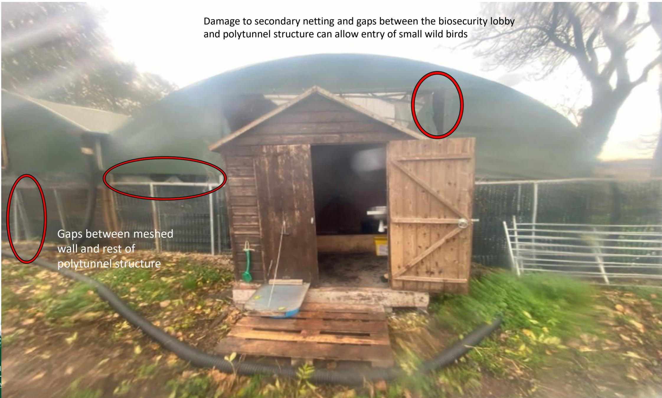
Gaps between meshed wall and rest of polytunnel structure
