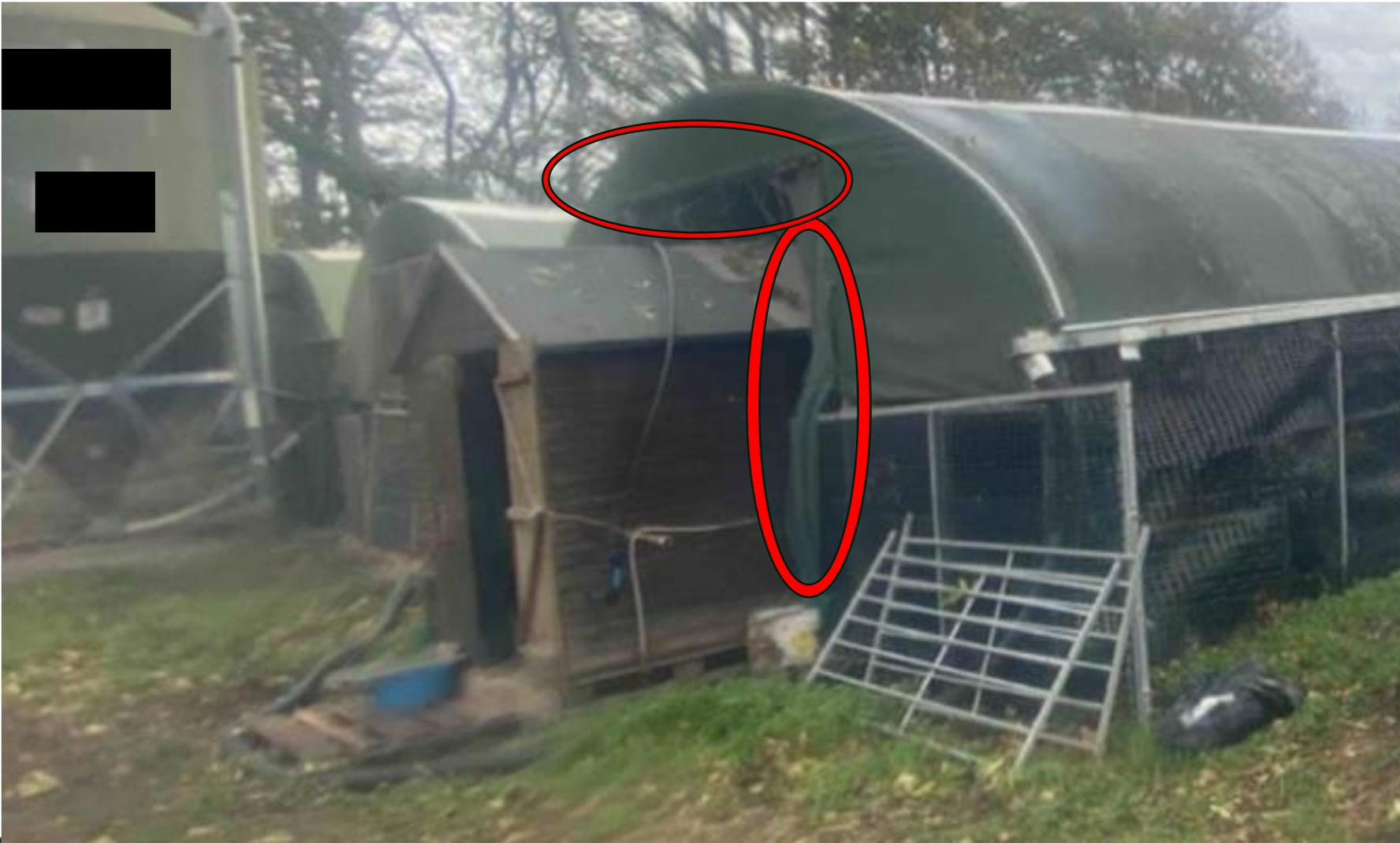
Apparent damage to secondary netting covering gaps between the biosecurity lobby and polytunnel structure can allow entry of small wild birds
